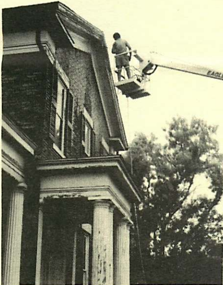
Using an aerial scaffold Bill Moore preps the wood trim before painting.
