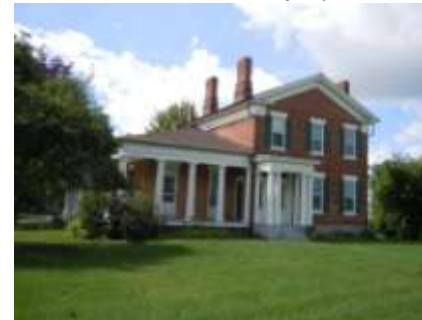
The Wisner House with newly replaced roof
