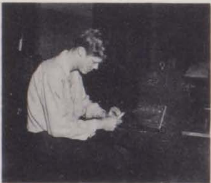
Transformer Testing — Electrical Shop
