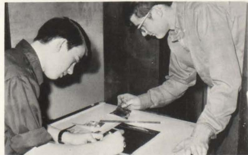
5. Roger Pelton and Mitchell Hensel are opaquing the negative that they have photographed from the dummy, in process for making a plate and printing it.
