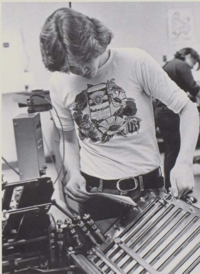
CARRYING OUT FINE ADJUSTMENTS, Scott Douglas sets the printing press before sending a piece of paper through on a trial run.
